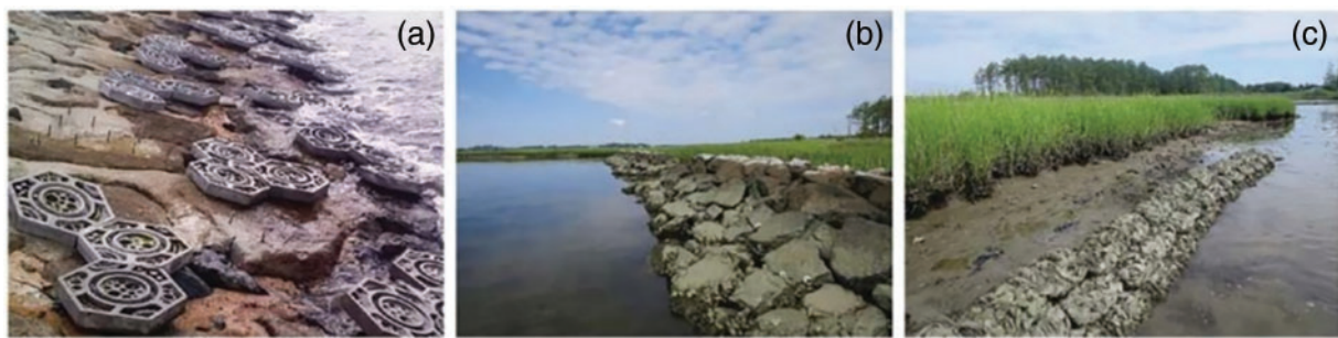
Fig. 4. Methods for eco-engineered shorelines (a) hard, (b) hybrid, and (c) soft, adapted from Morris et al. [51].
